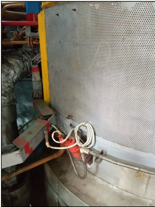
Figure 18: Flame Detector on Combustor Details
