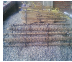
Fig 6: Caging of bamboo reinforced beams
