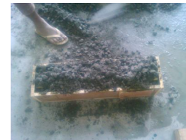
Fig 7: Concreting of bamboo reinforced beams.
