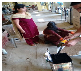
Fig 4: Providing bitumen coating on bamboo bars
