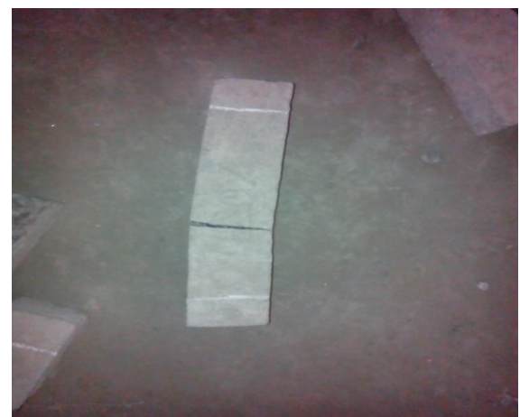
Figure 7: Cracking Pattern of Beam
