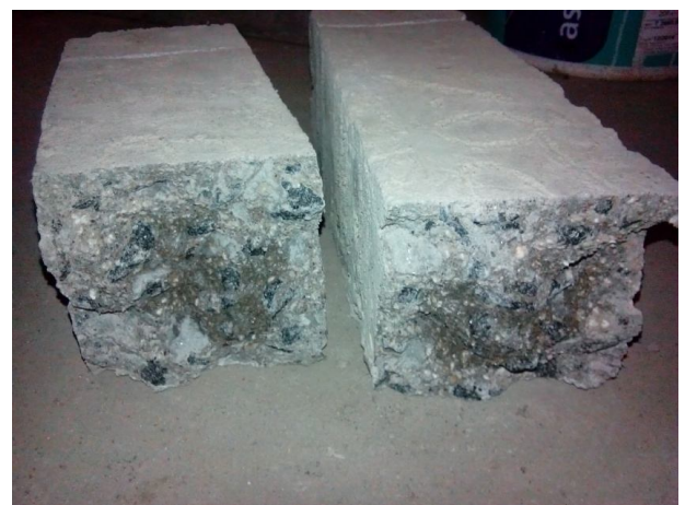
Figure 8 : Rupture of Beams
