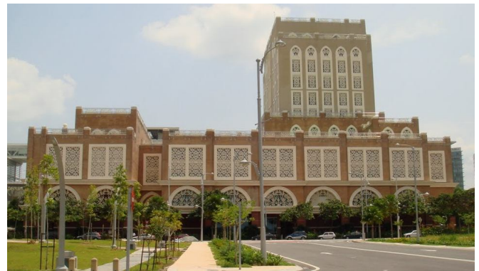
Figure 1: Building of Legal Affairs Section (LAS), Putrajaya, Malaysia.
