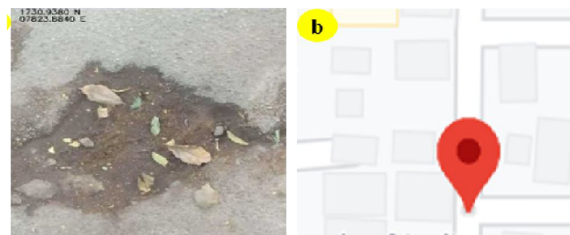
Figure 9: Location of pothole (a) Latitude and longitude values on pothole image (b) Detected pothole marked on google map.
