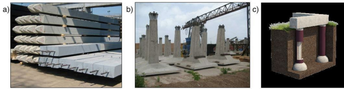
Figure 3: Construction and construction measures: a) piles covered with organosilicon enamel; b) foundations with a reverse slope and anchors; c) anchor piles according to the technology of individual construction and ecology (TISE) (compiled by the authors).
