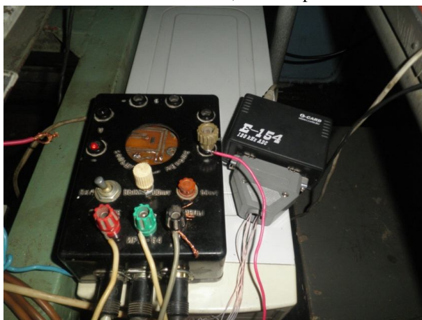
Figure 2,b. A general view of the power supply unit for Hall sensors and a digital converter E-154 for connecting to a computer is presented
