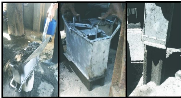
Figure 2: The casting of the mortarless interlocking hollow blocks
