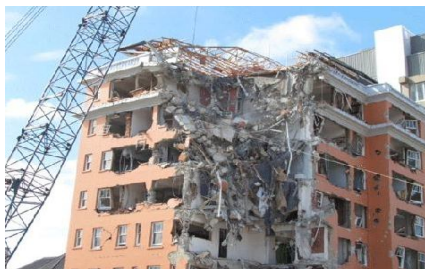
Figure 1: Demolition of the concrete buildings.
