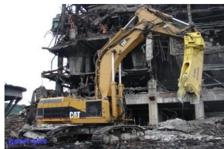
Figure 2: High precautions and requirements should be adopted during demolition's operations.
