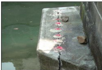
Figure 6: Bristar chemical using in demolition.
