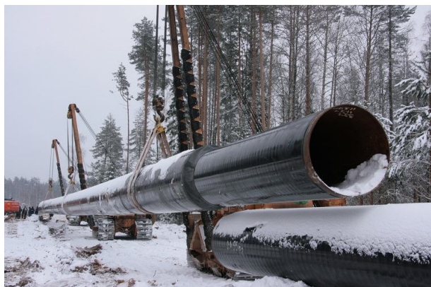
Figure 1: Construction of long-distance oil pipeline.
