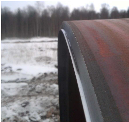
Figure 7: External view of pipe end preparation.
