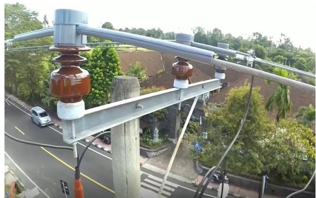
Figure 13: Isolator cap with electric shock to prevent animal walk closely.
