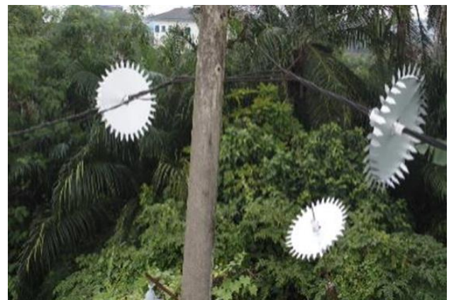
Figure 14: several type of animal crawling barrier (1).
