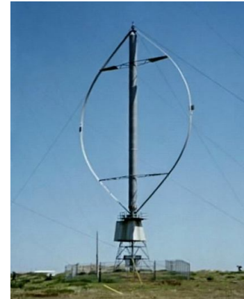
Figure 1: Darrieus wind turbine [1]
