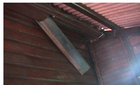
Figure 33: Broken ceiling
