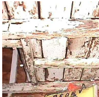
Figure 7(b): Decaying ceiling
