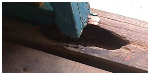
Figure 11: Rotted sill
