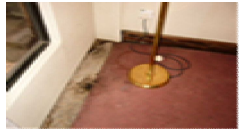
Figure 22: Having carpet material easily over run the glue and making the detachment process easily been done from the concrete floor slab of this office space
