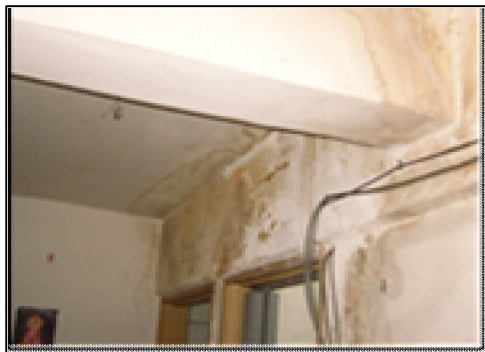
Figure 42: Anti-fungus coating is being applied for this rectification work of an interior space. The task requires expert personnel to ensure the space back to its original condition and in reusable state
