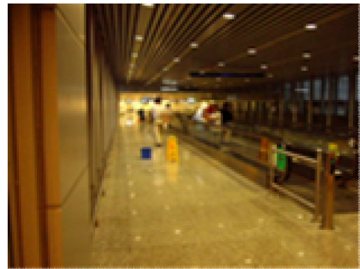
Figure 9: The photograph shows plastic pail has to be located at the spots where the water leakage, this one next to walkalator linking parking to terminal building
