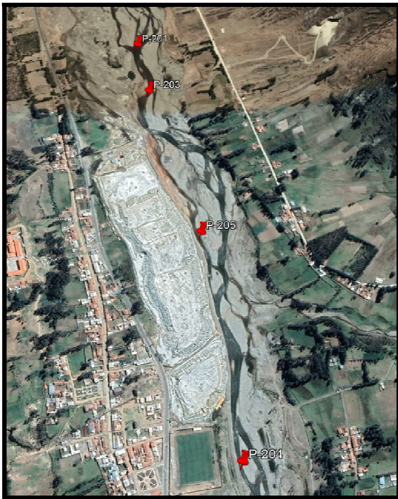
Figure 2: Ticapampa’s environmental liability and Santa River
