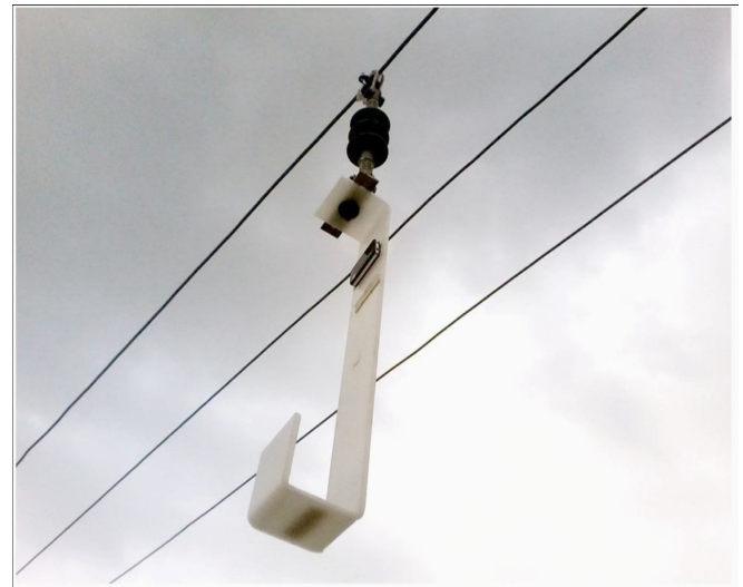
Figure 2: Field test conducted at mid span
