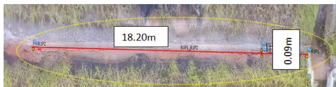
Figure 10: Damage Analysis of 3D models Crack No 2
