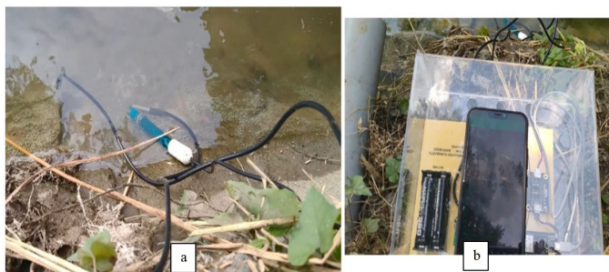
Figure 11: Transmitter Installation at the River Bank During Field Testing: a) the Three Sensors are Exposed to the River Water, and b) the Transmitter Box with Smartphone Just to Show the Exact Coordinate in the Map
