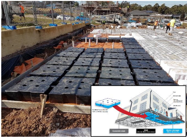
Figure 1: Types of individual lot stormwater detention system using a) Precast concrete and b) Polyethylene [3,4].
