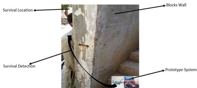
Figure 11. Block structure Material System Testing
