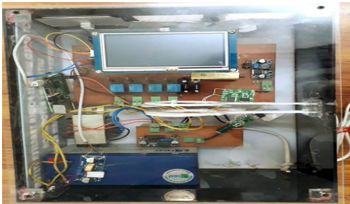
Figure 14: Outside view of wireless power transfer based home automation
