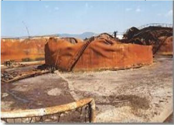
**Figure 2.1: Damaged Liquid Storage tank (A) due to sloshing**
