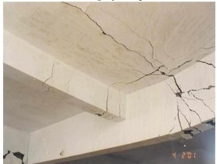
**Figure 2.5 : The beams of ground floor roofs were heavily damaged due to fall of filled water tank from the roof of the adjacent building.**
