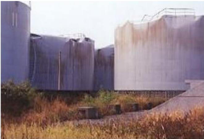
**Figure 2.2: Damaged Liquid Storage tank (B) due to sloshing**
