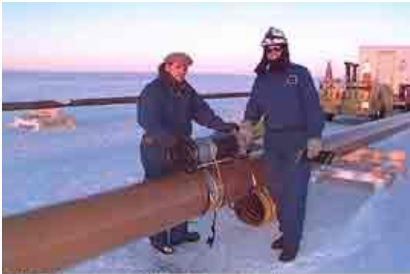
Photo Courtesy of Yxlon International
