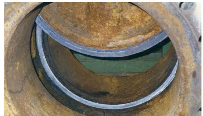
Figure 10: Reconditioning of wedge gate
