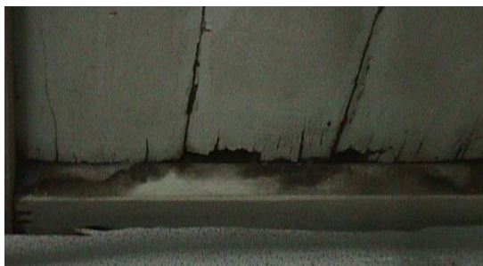
Figure 19(a): Dirty wood panelling
