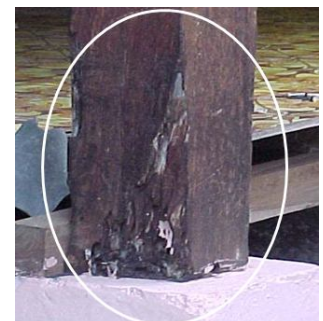
Figure 20(b): Rotted pillar
