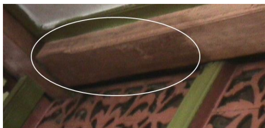
Figure 27(a): Dirty roof beam
