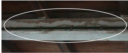
Figure 6(b): Water stains on roof beam
