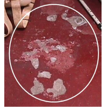
Figure 24(d): Potholed surface
