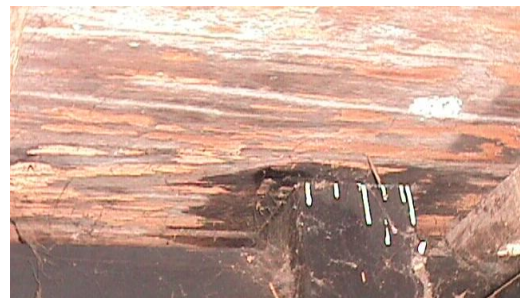
Figure 11(b): Rotted floor
