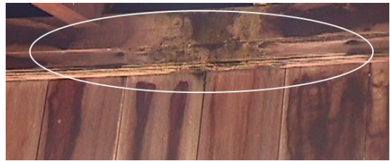
Figure 27(b): Faded colour of wooden roof beam
