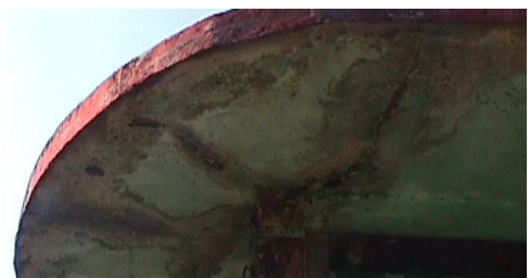
Figure 30(a): Water stains on concrete roof
