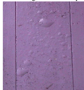
Figure 15(a): Bulging paint
