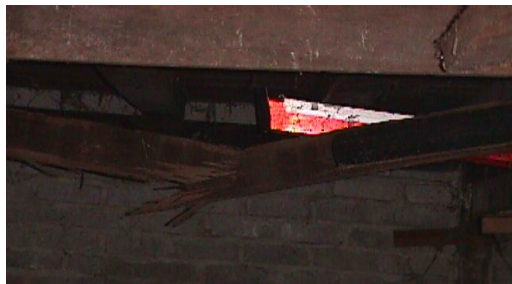
Figure 2(b): Broken floor girders
