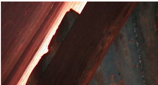
Figure 7(b): Rotted main rafter
