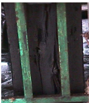
Figure 14(a): Decayed pillar
