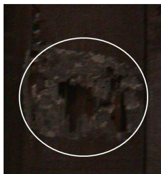
Figure 14(b): Decayed pillar
