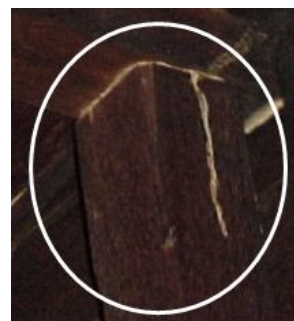
Figure 20(a): Rotted pillar
