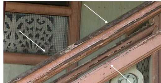
Figure 33: Peeling paint finishes
