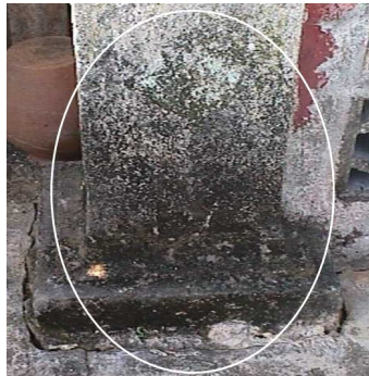
Figure 26(b): Dirty pillar surfaces
