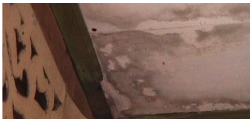
Figure 31(a): Water stains on ceiling
