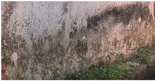
Figure 25(d): Dirty wall surface
