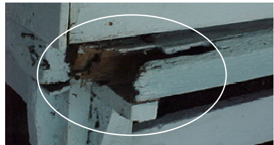
Figure 5(a): Rotted sill
