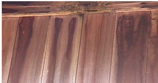
Figure 25(e): Faded timber colour
