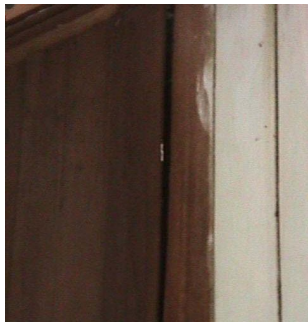
Figure 13(a): Ruptured wall
