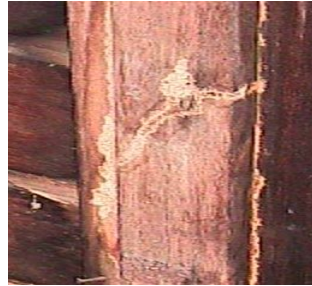
Figure 21(b): Decayed frame
