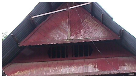
Figure 16(b): Faded paint surface
