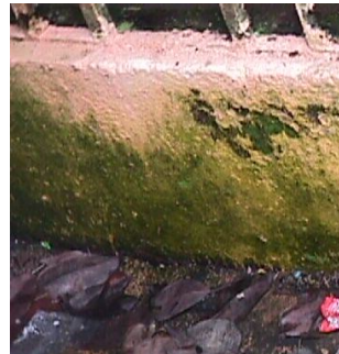
Figure 13(b): Mossy brick wall
