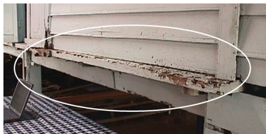
Figure 5(b): Rotted sill
