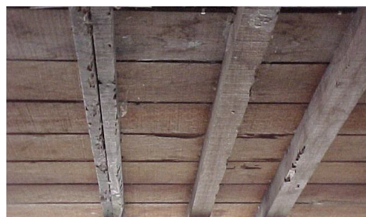
Figure 12(a): Rotted floor girders
