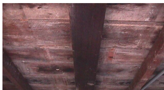
Figure 1(b): Faded wood surface colour
