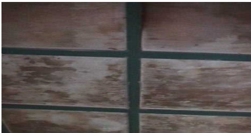
Figure 31(b): Mosses on ceiling
