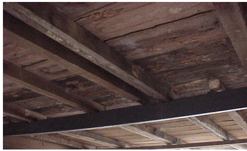
Figure 12(b): Destroyed girders and floor boards
