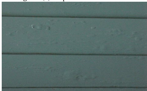
Figure 3(b): Bulging paint surface
