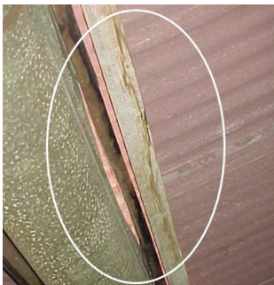
Figure 22(c): Leaking rain gutter
