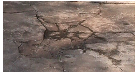
Figure 24(b): Cracked floor apron
