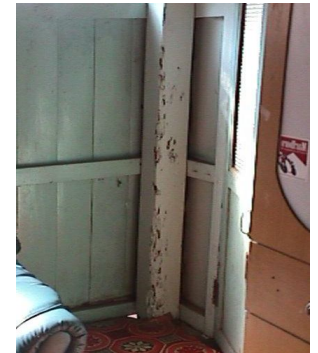
Figure 4(b): Rotted pillar
