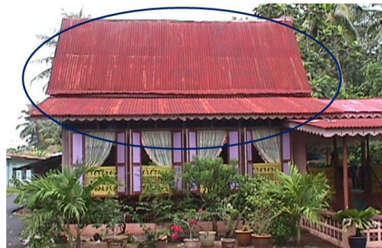
Figure 16(a): Rusted zinc roof
