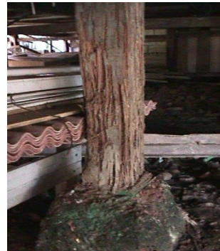
Figure 4(a): Rotted pillar
