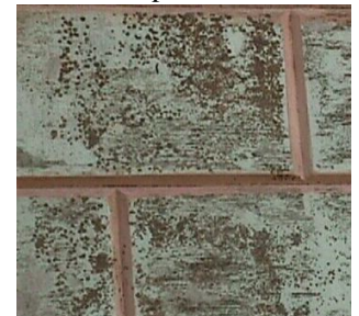
Figure 25(b): Peeling paint
