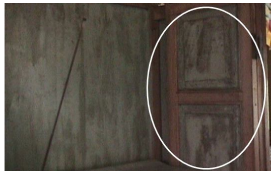
Figure 29: Dirty door surface
