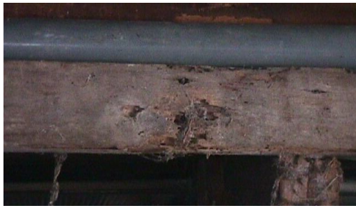
Figure 2(a): Rotted floor girders
