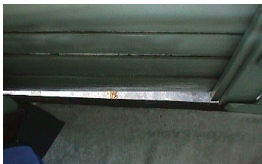
Figure 3(a): Gap between floor and wall
