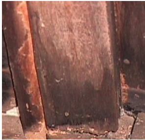
Figure 21(a): Faded paint
