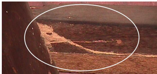
Figure 22(a): Destroyed rafter connections
