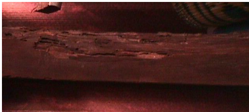
Figure 7(a): Damaged roof rafter
