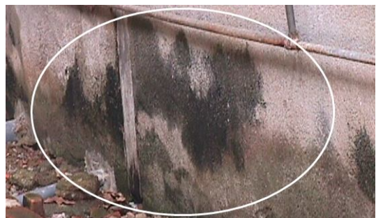
Figure 19(e): Stains on wall
