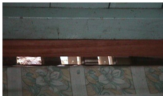
Figure 1(a): Untidy floor joining
