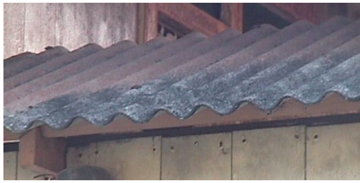
Figure 30(b): Dirty roof finishes
