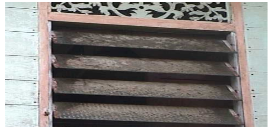
Figure 28: Dirty window surface
