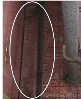
Figure 24(c): Faded floor
