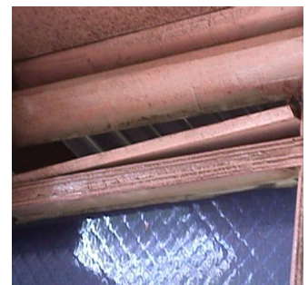
Figure 15(b): Broken timber
