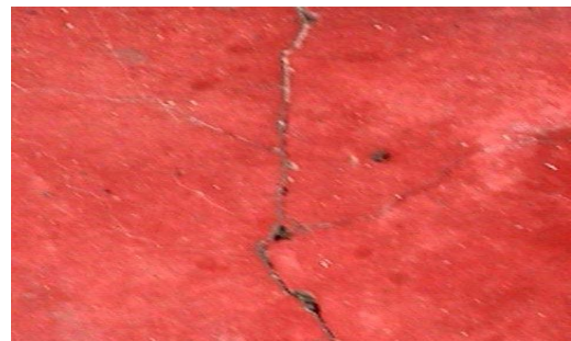
Figure 11(a): Cracked floor apron
