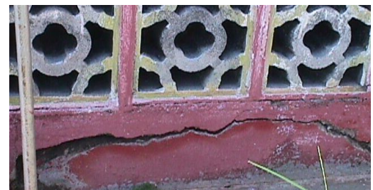
Figure 25(c): Cracked wall surface
