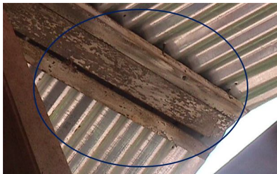
Figure 16(d): Peeling wood surface
