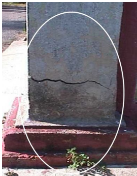
Figure 26(a): Cracked pillar
