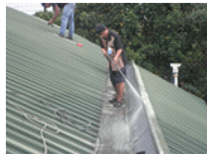
Figure 16: Leakage at joints of metal gutter
