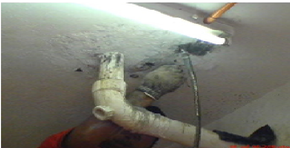
Figure 14: Grouting process method being done
