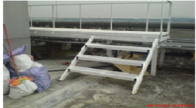
Figure 9: Leaking on the surface of the concrete flat roof
