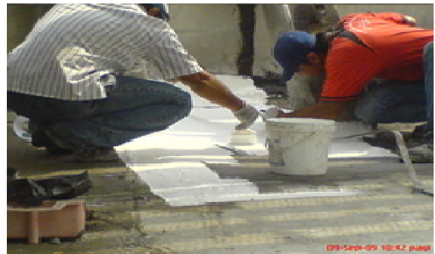
Figure 10: Rectification done by applying cementitious epoxy coatings
