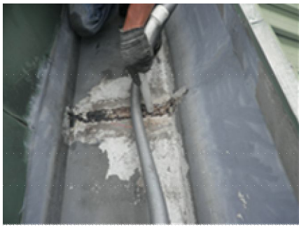
Figure 17: Replacing the epoxy at the joint being done
