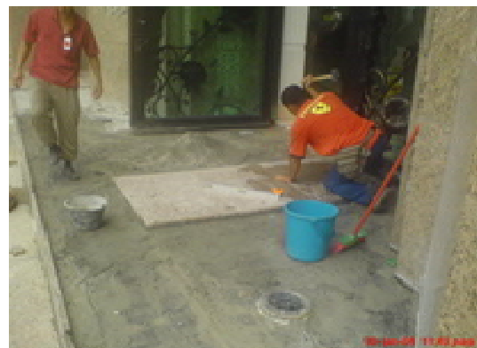
Figure 11: Exterior marble floor replacement
