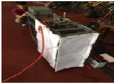
Figure 10: Installation sound absorbent at MGT
