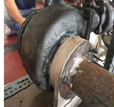
Figure 6: Back View of Turbines
